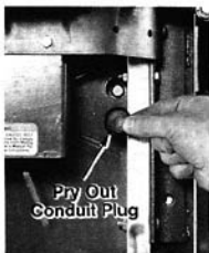
(Photo 5-18) Pry out conduit plug with a screwdriver.
