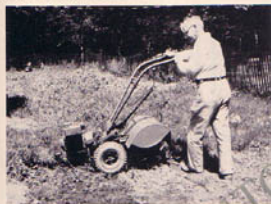
(Photo 5/6B) Swing handlebars around.
