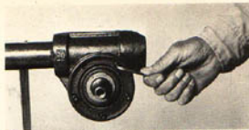
(Photo 8/11) Remove tiller housing cover screws.
