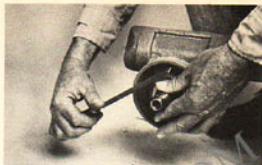
(Photo 8/138) Remove nicks and install lines.
