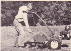
(Photo 5/2) Wheel speed select lever
