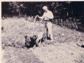
(Photo 5/6C) Let wheels drive tiller in furrows.
