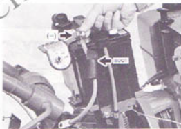
(Photo 37) Connect negative (-) cable to negative (-) battery post. Then cover post with rubber boot.
